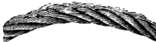
Wear caused by a damaged drum.
